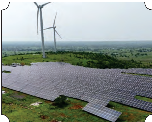
IREDA funded 2.3 MW Solar PM-KUSUM project in Shajapur, Madhya Pradesh
