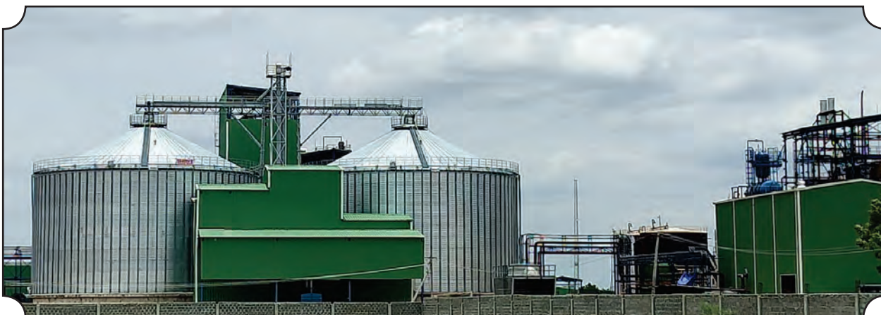
IREDA funded 120 KLPD Ethanol project located in Telangana, developed by Whitefield Bio Products Pvt. Ltd.
