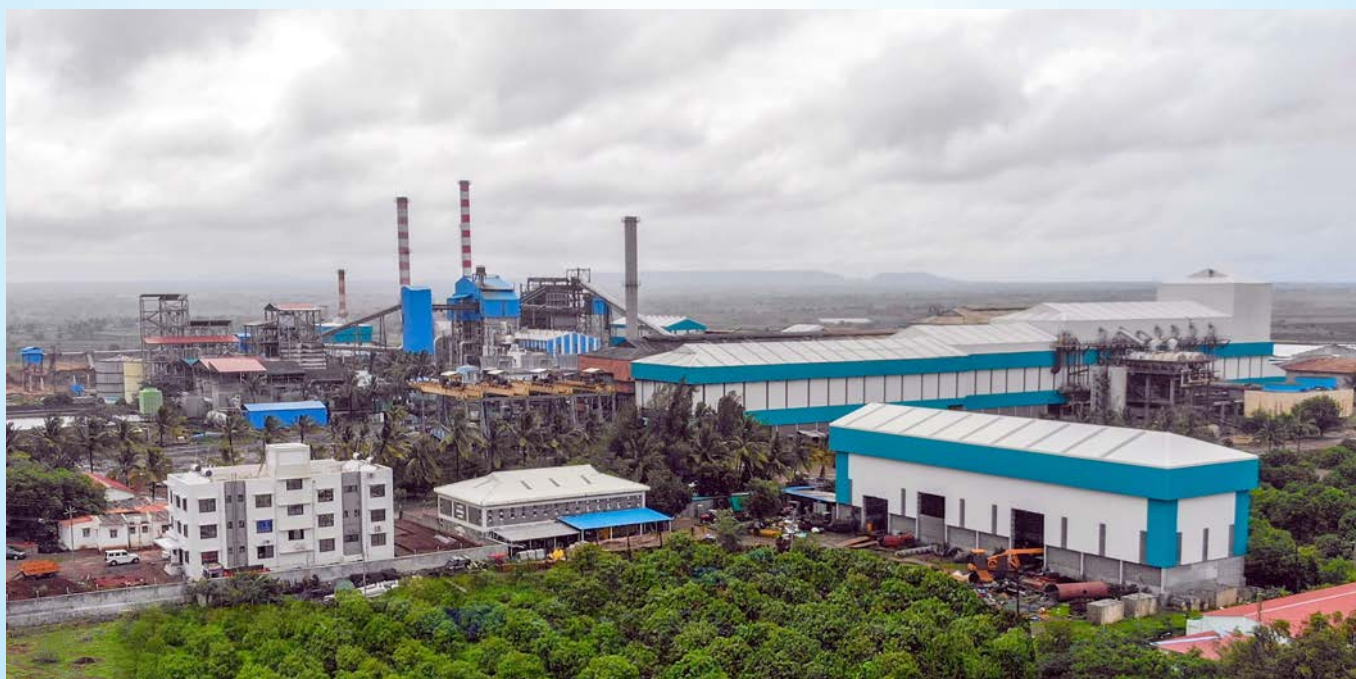
IREDA financed 28 MW Bagasse Based Cogeneration Project situated at Village Vishnuannanagar, Post Navalihal, Taluk Athani, District Belagavi, Karnataka
