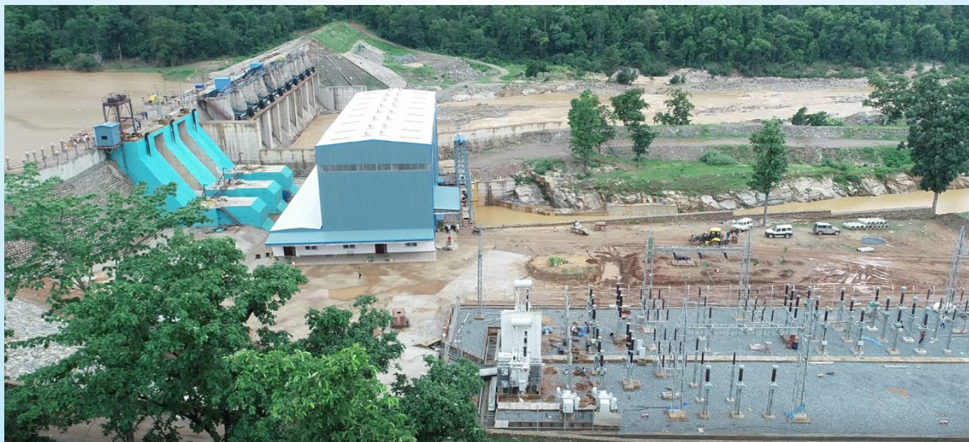
IREDA funded 24.75MW Mahan-III Hydro Energy Project at Chikni Village, Surajpur District, Chhattisgarh
