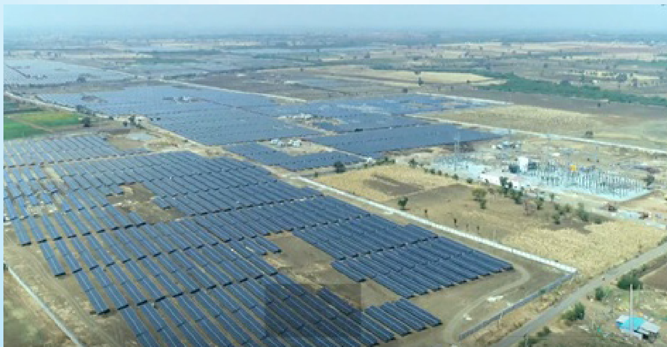
IREDA funded 135 MW Solar Project located at Kurthakoti Village, Gadag District, Karnataka
